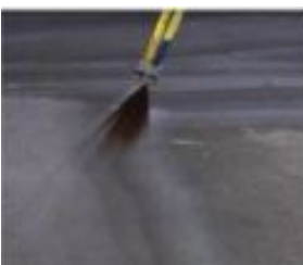
Picture: Spray Grade being applied.
