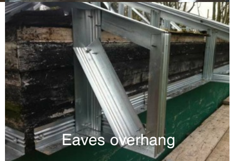
Main frames installed
