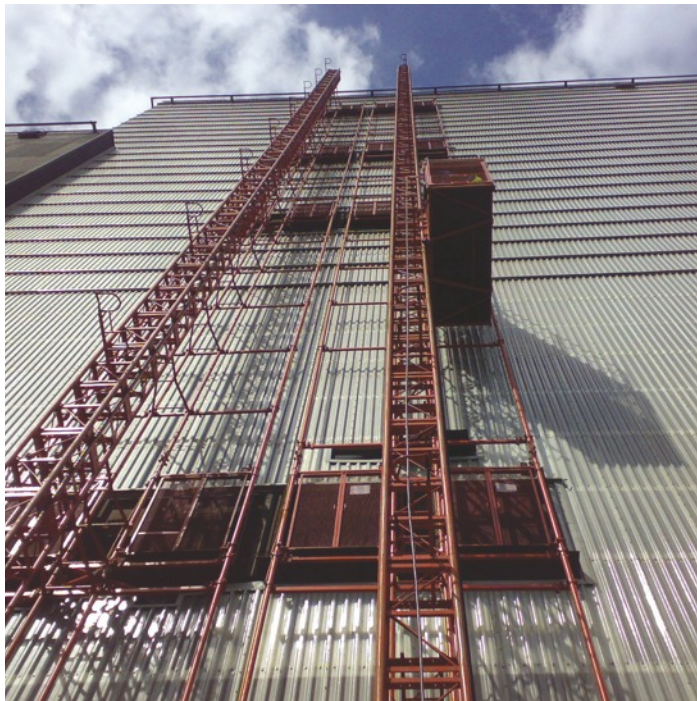
Power station cladding
