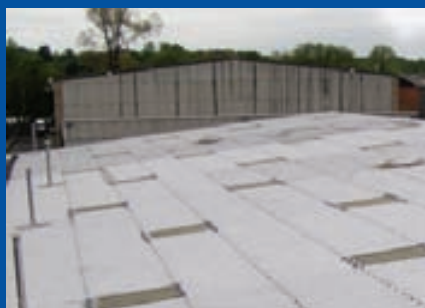
A factory roof in Camberley, Surrey, before and after refurbishment with FILON over-roofing
