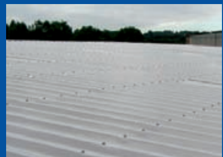
A factory roof in Camberley, Surrey, before and after refurbishment with FILON over-roofing
